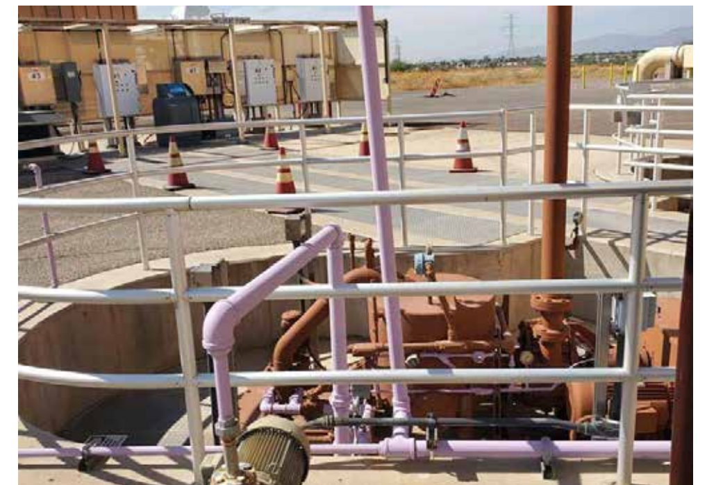
Grit Chamber, grit pump and grit seal water pump: The grit chamber primary catches inorganic solids such as sand, gravel, glass, corn, and soil.
