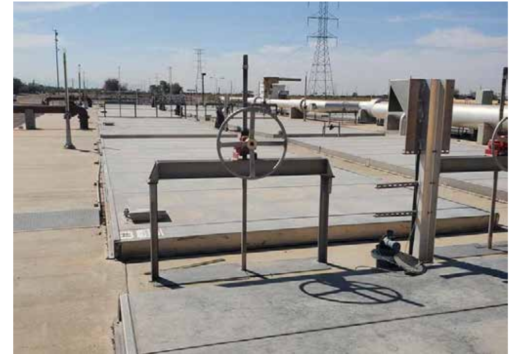
Aeration Basin Flow Control Gate controls the pressure and flow of air for treatment ponds and promotes biochemical oxidation of wastewaters.
