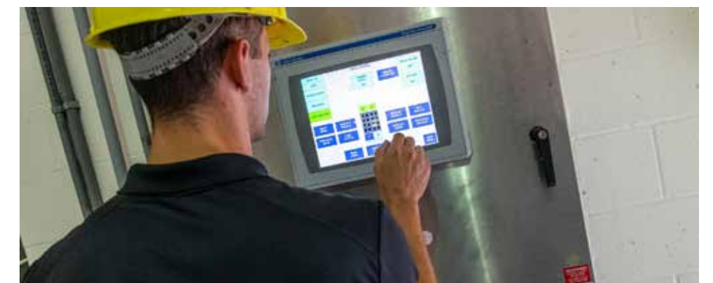
Callahan checks the status of the TrojanUV4000Plus (TrojanUV) disinfection system.
