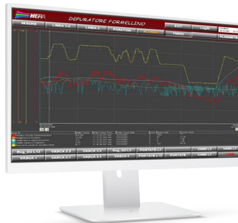
Intuitive displays show the plant status to operators at any given time.
